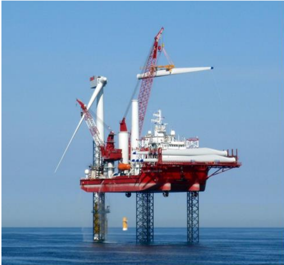
Figure 3: Seajacks Leviathan vessel
