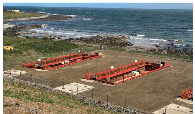
Typical landfall compound with two Transition Joint Bays
